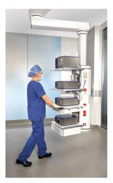
Endoscopy workstation: dual mechanical Moduevo Beam with Mezzo Distributor
