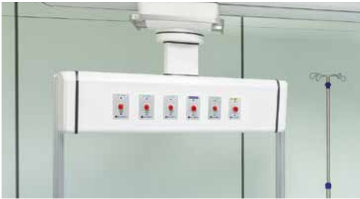
Three panels for outlets and sockets (including underneath).
